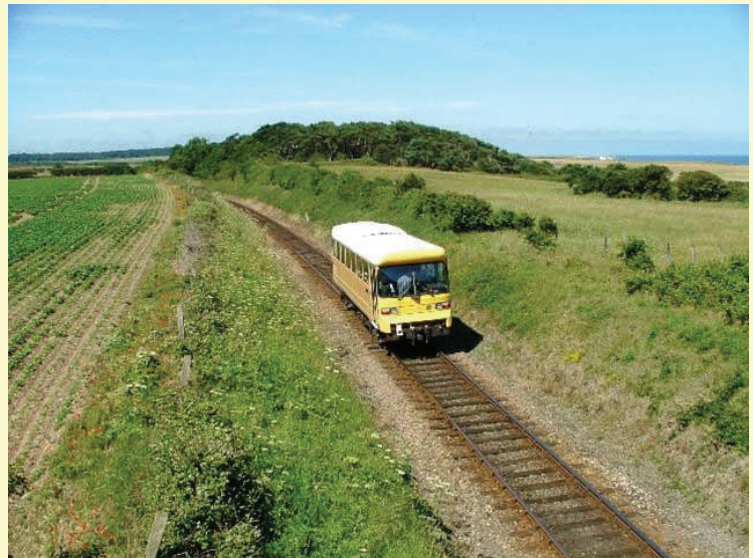
LEV1 passing Dead Man's Bridge working from Sheringham-Holt during the Diesel Gala
